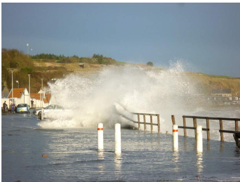
Overtopping of stepped revetment at Cowie promenade. Photograph supplied by Aberdeenshire Council.
