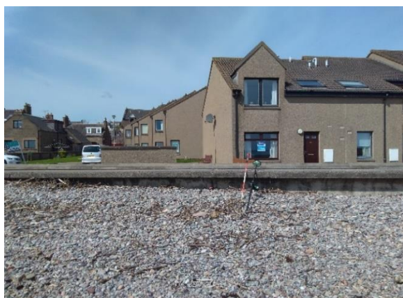
Figure 3-8: Section C/XS17: Seawall with sediment build up and shingle beach
