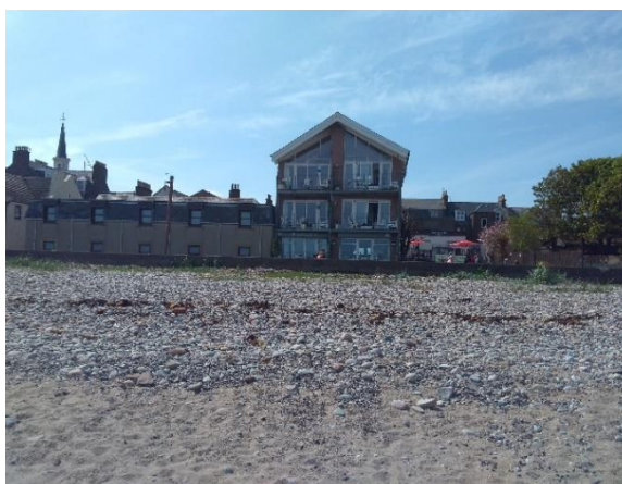
Figure 3-9: Section D/XS20: Seawall with sediment build up. Shingle and coarse sand beach.
