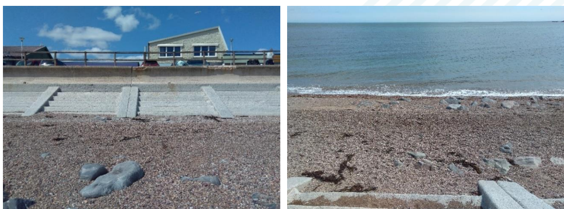
Figure 3-6: Section B/XS12: Stepped revetment and shingle beach
