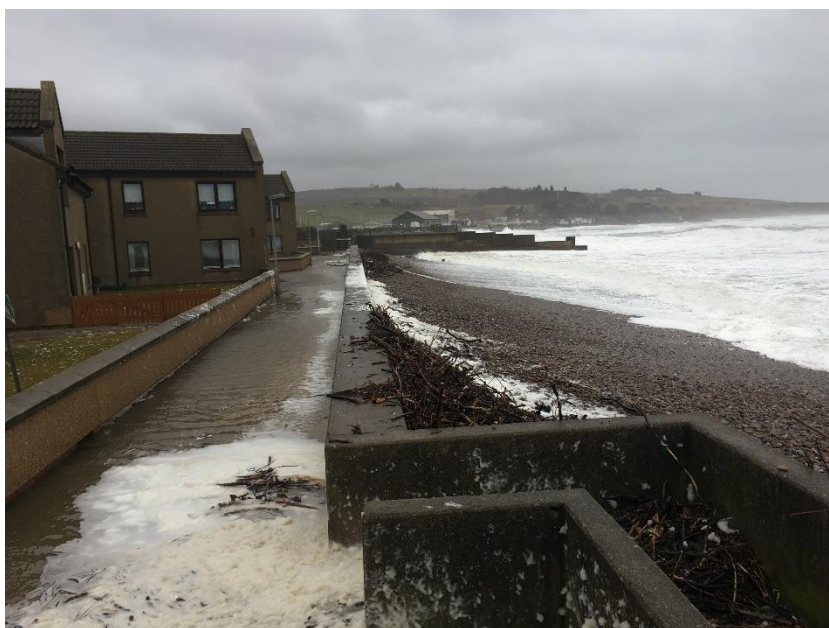
Overtopping of central wall section. Photograph supplied by Aberdeenshire Council.
